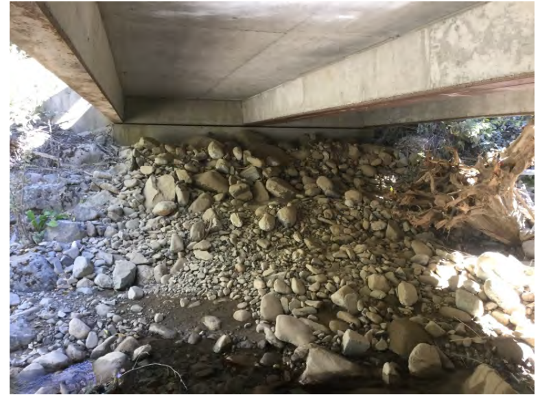
Right Bank Abutment when facing downstream
