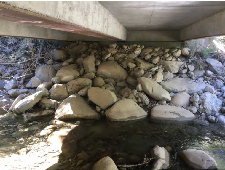
Left Bank Abutment when facing downstream
